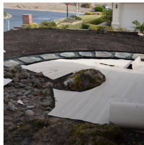
During the Transformation
